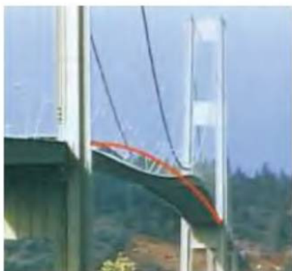
This photograph shows the Tacoma Narrows suspension bridge on the day in 1940 when it experienced a wind-induced standing-wave oscillation that led to its collapse. The red line shows the original line of the deck of the bridge. You can clearly see the large amplitude of the oscillation and the node at the center of the span.
